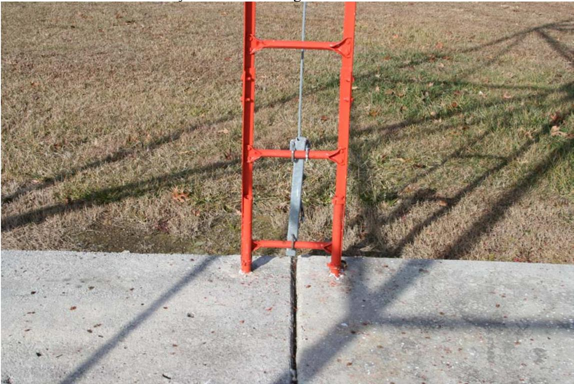
Another detail view of the Crossville, TN airport beacon tower showing the tubular base for the ladder attachment.
